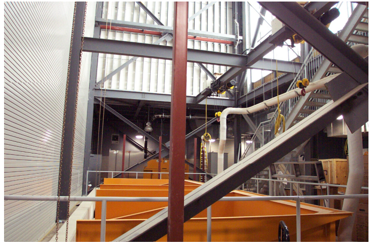
Figure 5. Example of Indoor Cake Receiving Station at GEB WWTP
