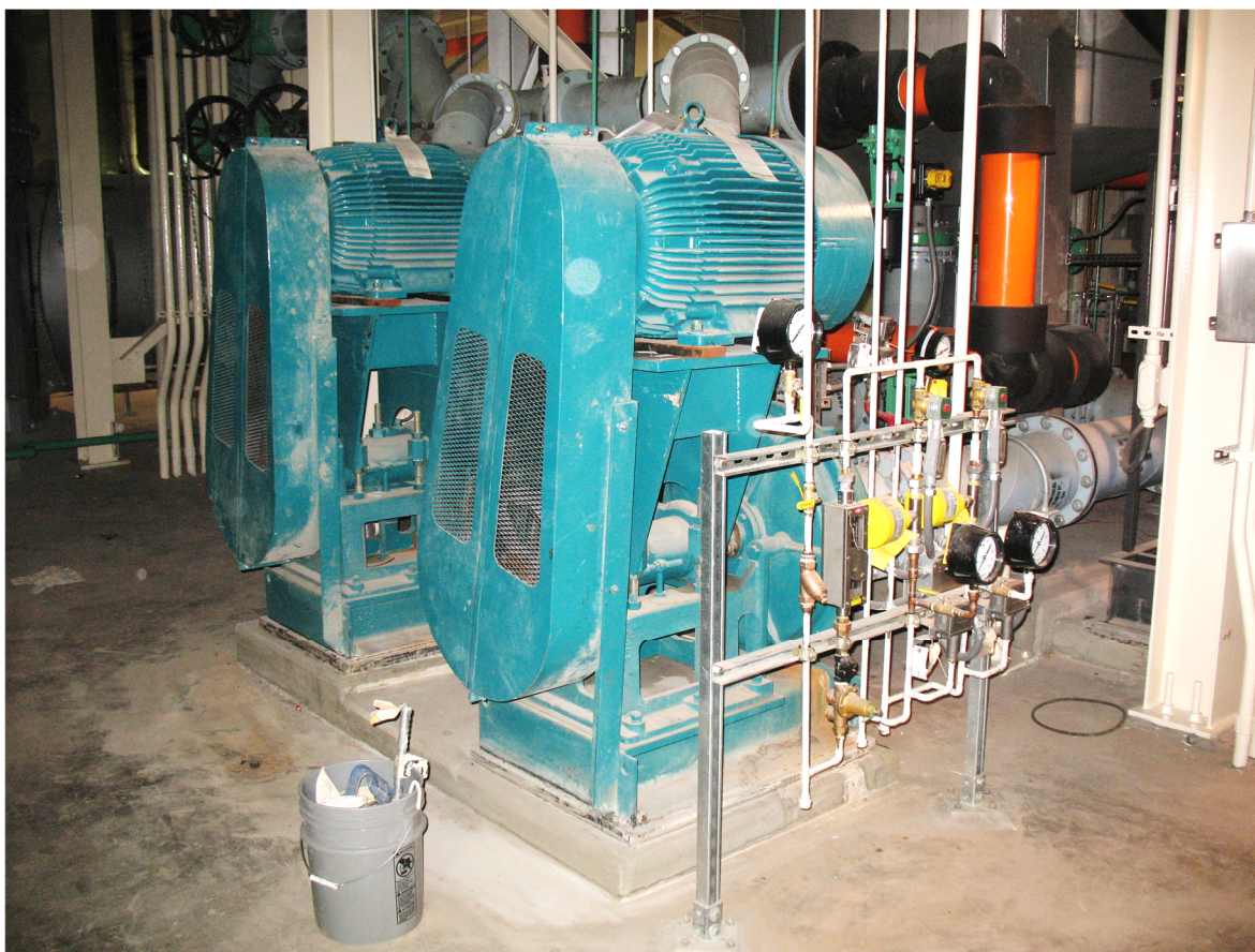
Figure 4-3. Example Installation of Ash Slurry Pumps Installed Directly to Wet Scrubber Drain Outlet
