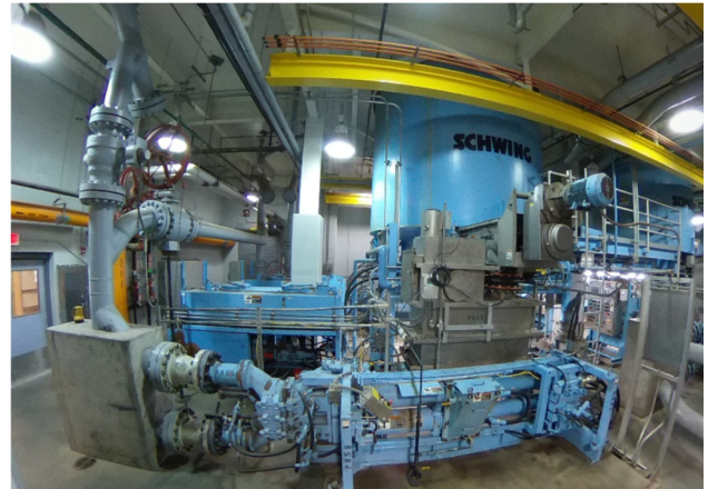
Figure 10. Dual-Piston Hydraulic Cake Pump Paired to a Sliding Frame Bin at MCES' Metro WWTP
