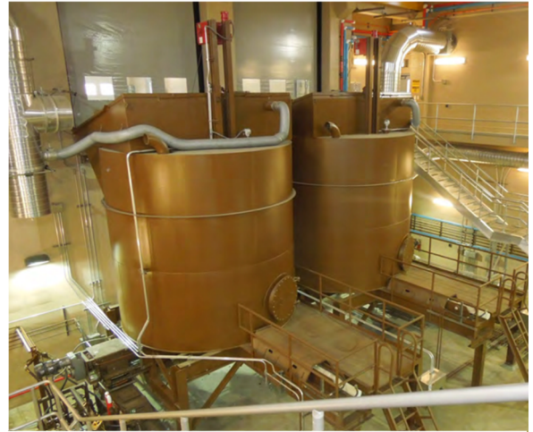
Figure 7. Below Grade Cake Receiving Bins Designed for Maximum O&M Access
