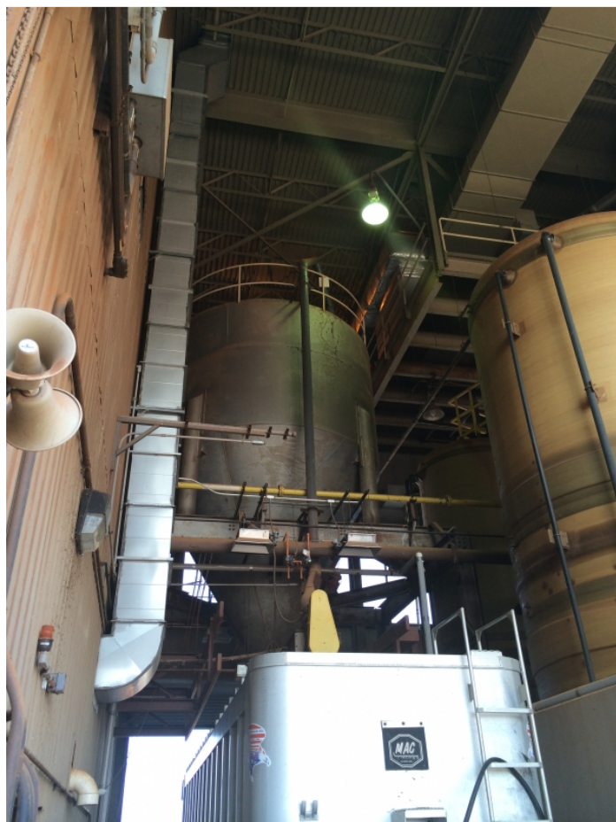
Figure 4-11. Example Dry Ash Loadout Facility (Indoor)
