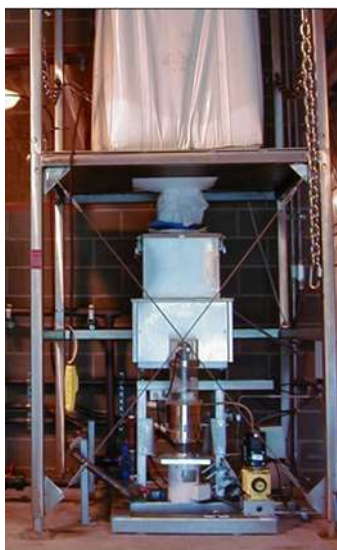
Figure 4-10. Dry Polymer Feeder with Bulk Bag Frame
