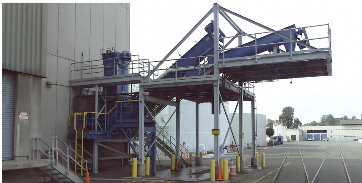
Figure 4-10. Example Dry Ash Loadout Facility (Outdoor)
