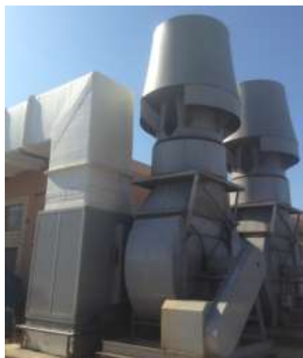
Figure 5-2. High-Velocity Exhaust Fans Used for dispersing low-concentration room air
