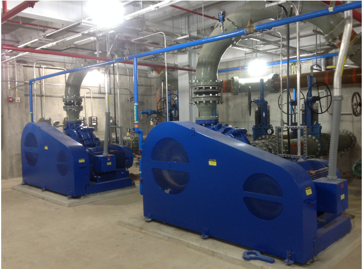
Figure 4-6. Example Installation of Ash Slurry Pumps Downstream of Ash Slurry Tanks
