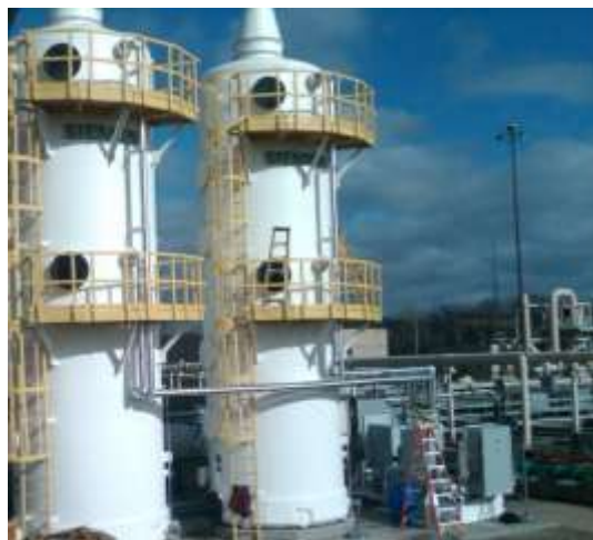
Figure 5-4. Biotrickling Filters
