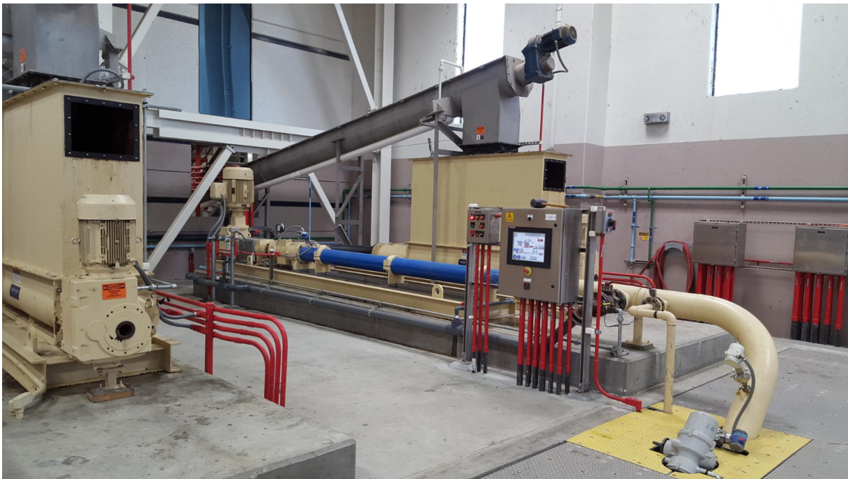
Figure 3. Example of Multi-Stage Progressing Cavity Pumps for Dewatered Sludge Cake
