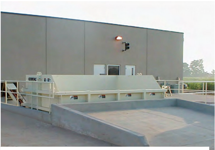
Figure 4. Example of Outdoor Cake Receiving Facility (Photo Provided by Schwing Bioset)
