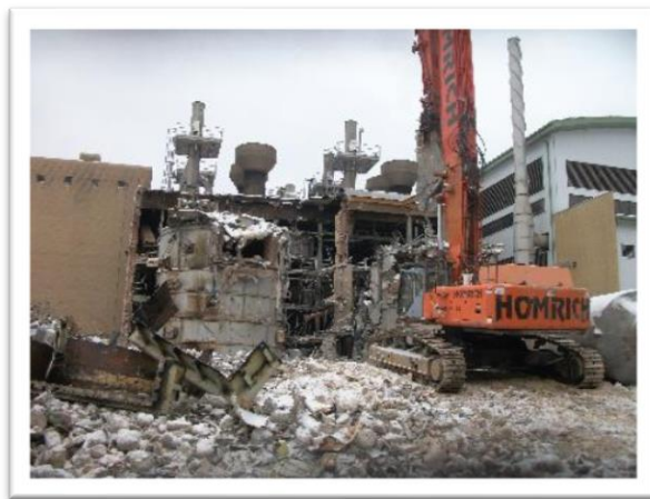
Figures 3-1 and 3-2: Demolition of MHI facilities at the Cincinnati Mill Creek Wastewater Facility.
