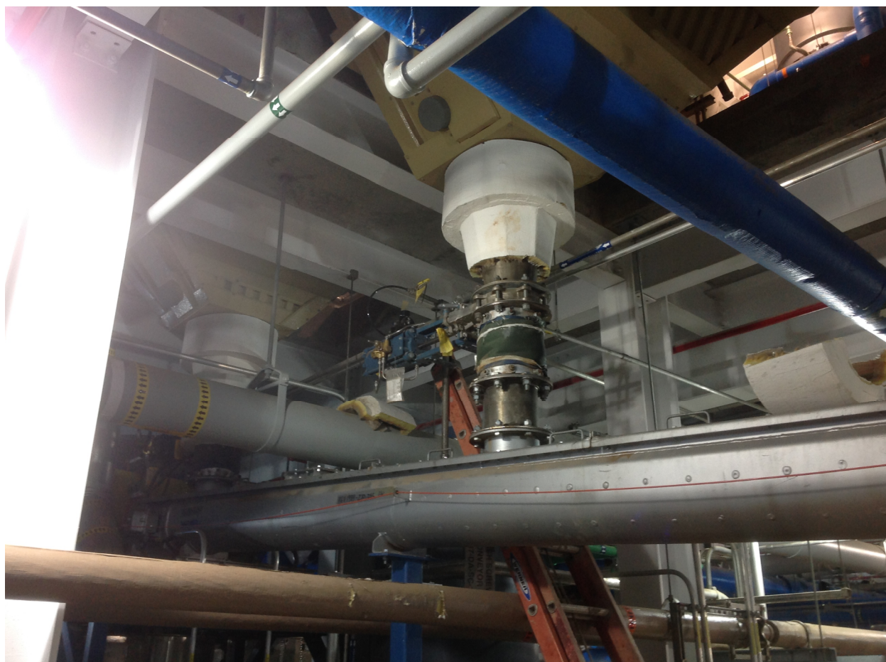
Figure 4-4. Example Boiler Ash Discharge Approach
