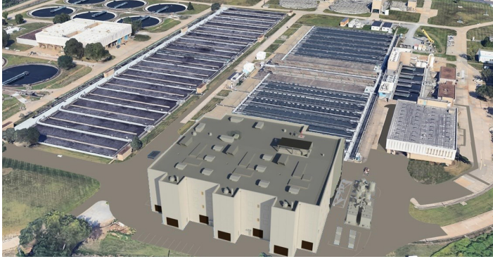
Lemay Wastewater Treatment Plant: Rendering of completed Solids Processing Building. No smoke stacks!
