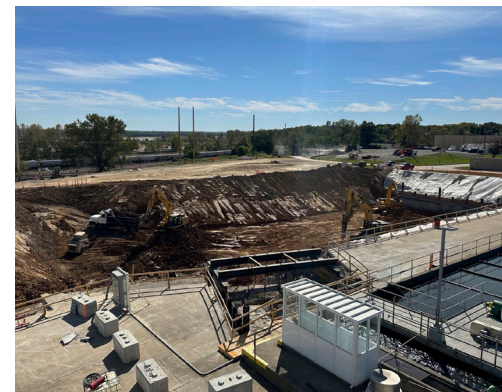
Lemay Wastewater Treatment Plant, October 2024: Solids Processing Building (SPB) basement and interconnecting tunnel excavation.
