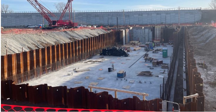
Bissell - Basement concrete construction in progress
