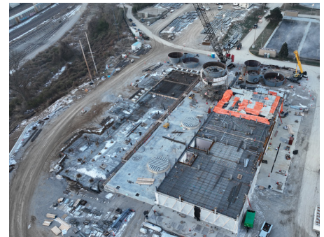
Drone view of the Lemay SPB: orange thermal blankets cover newly placed concrete, scaffolded reactors stand at center, and steel columns outline the future superstructure.
