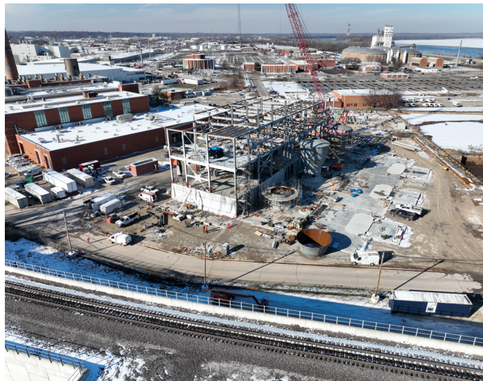
Structural-steel framing has topped out on the dewatering side of the SPB, while the first incinerator reactors take shape below, captured here in a snowy December 2025.
