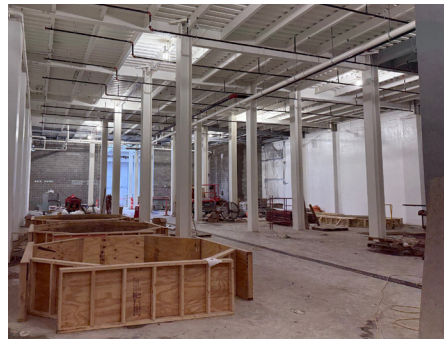
Inside the dewatering side of the SPB: freshly painted columns, completed raised slab decking, and formwork for equipment pads signal that interior fit-out is moving forward.
