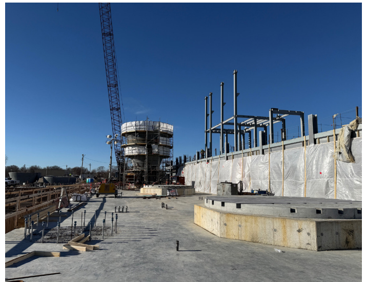
At Lemay, crews erect the first reactor while steel rises on the incinerator side of the SPB; heated sheeting protects winter concrete work along the foundation.
