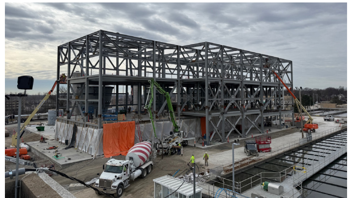
Structural steel framing advances on the Lemay SPB, with ongoing concrete work and equipment coordination below.
