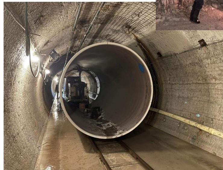
Jefferson Barracks Tunnel
