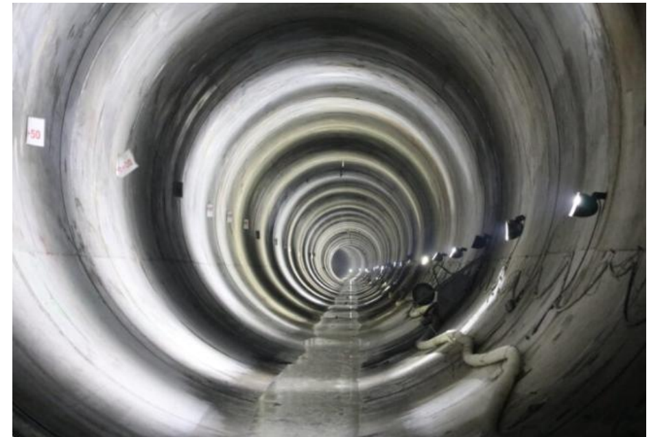
Deer Creek Tunnel, lining installed.
