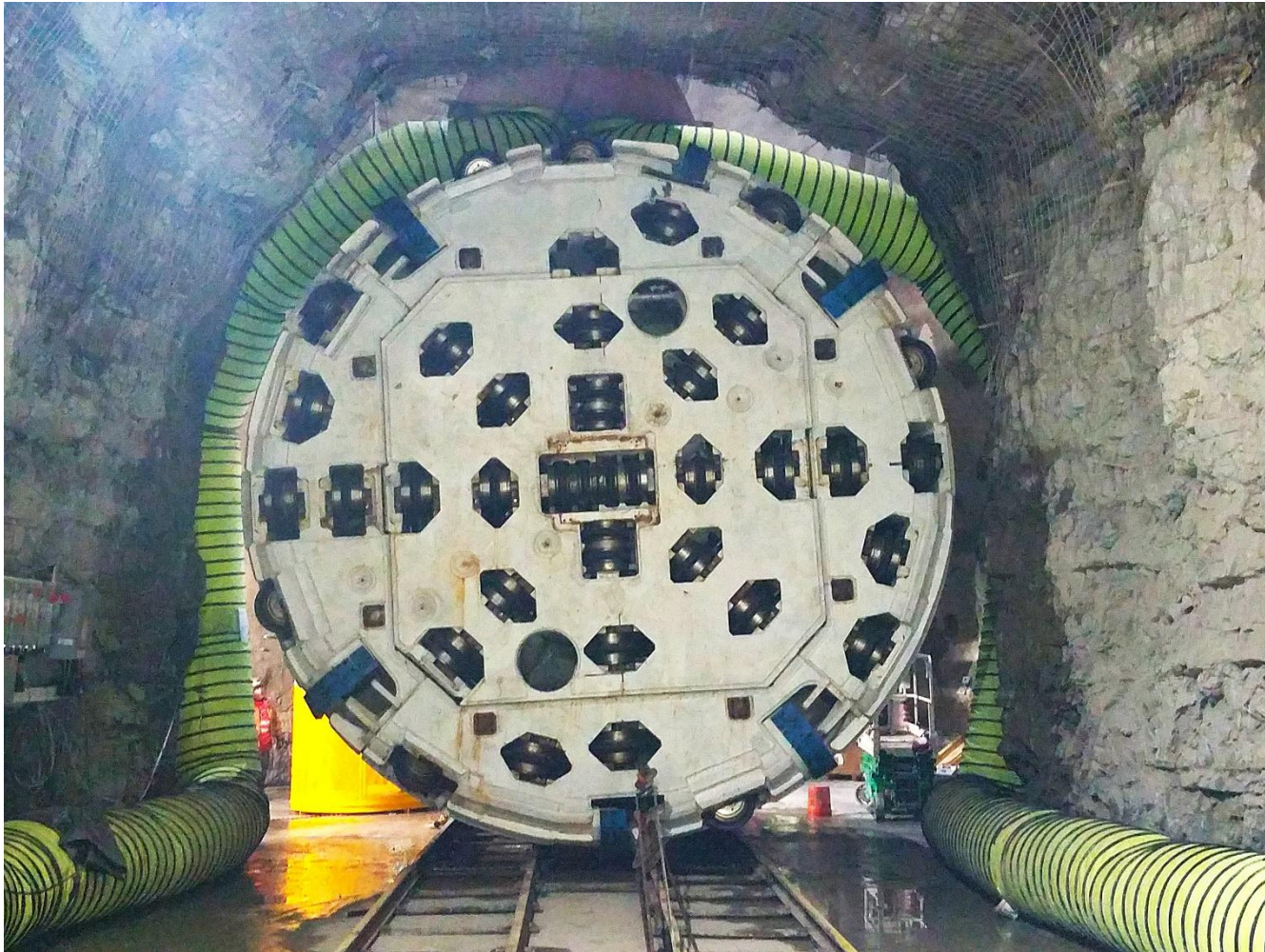
Deer Creek Tunnel, Main Beam TBM.
