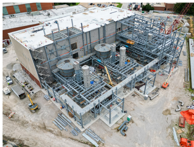
Above: Aerial view of structural steel erection, process equipment, and platform framing progress at the Bissell SPB.
