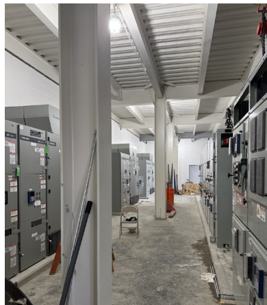
Medium voltage electrical distribution equipment installed in the Lemay SPB.
