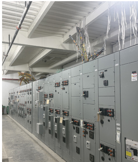
Electrical distribution equipment installed in the Lemay SPB.
