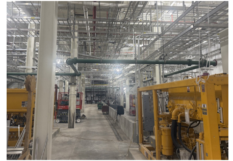
Process piping, cable tray, and equipment installation in the Bissell SPB basement.
