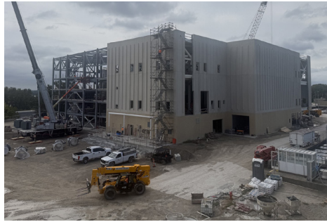
Precast wall panels and structural steel framing progress at the Lemay SPB.
